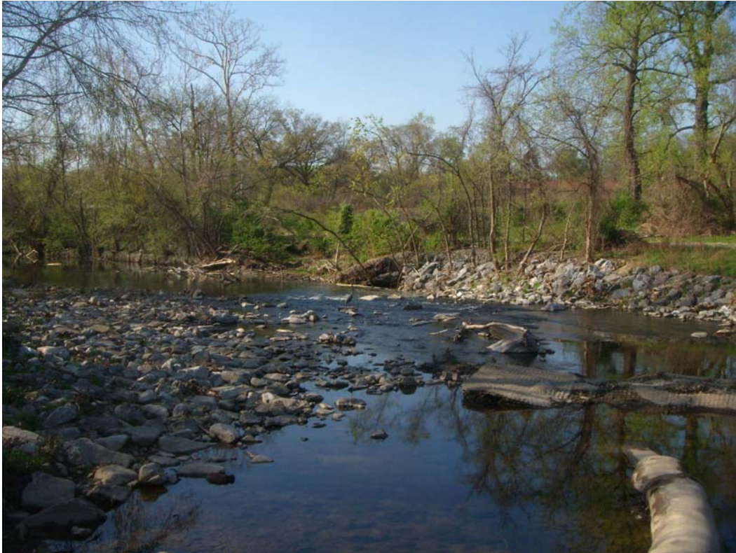
Northwest Branch– 5 looking downstream, April 2008
