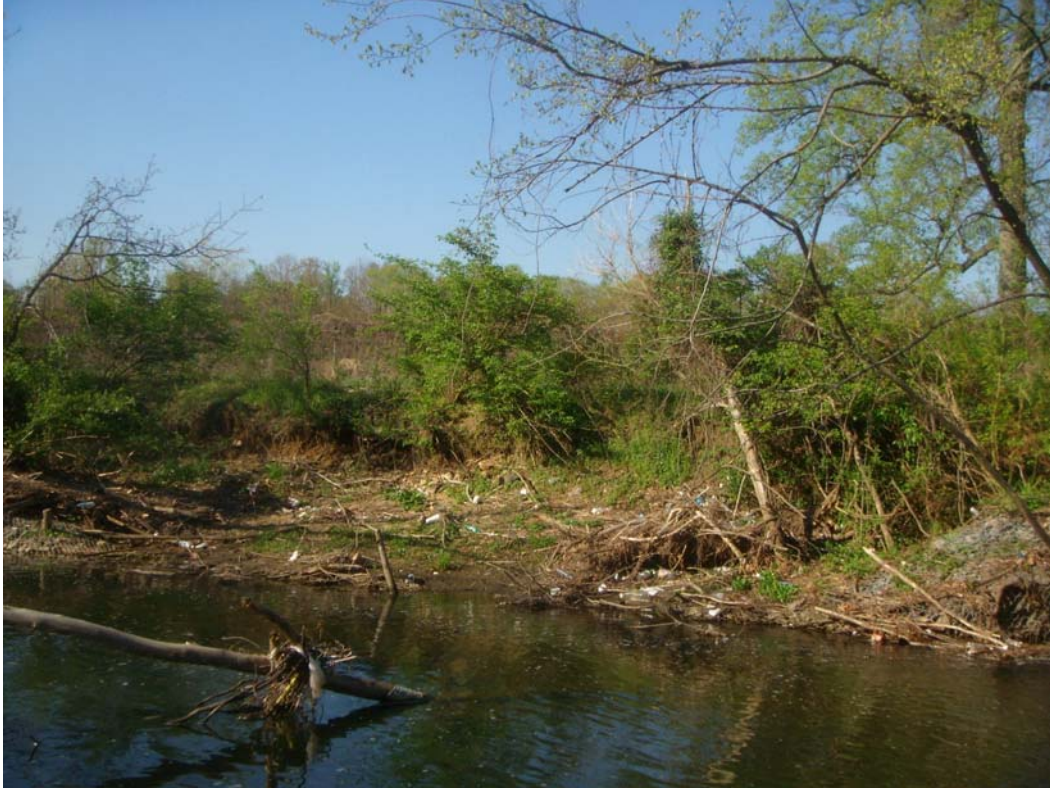
Northwest Branch – 5 Collapsed gabion and bank, April 2008
