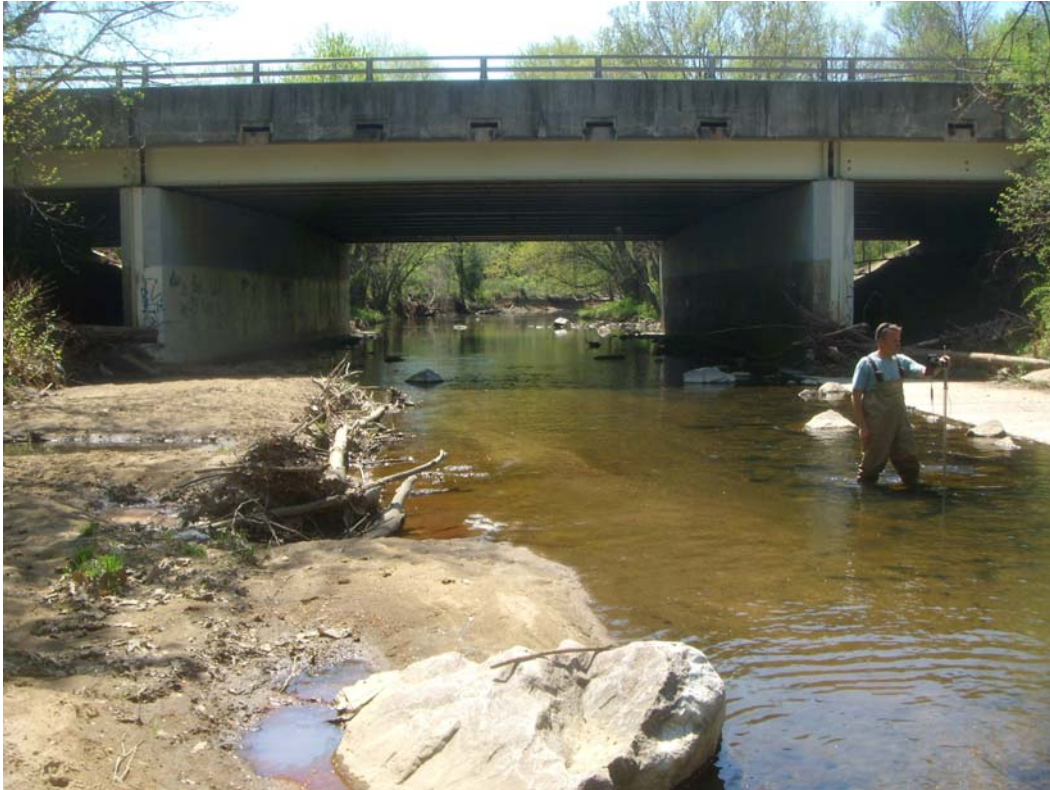
Northwest Branch – 8 looking downstream, April 2008
