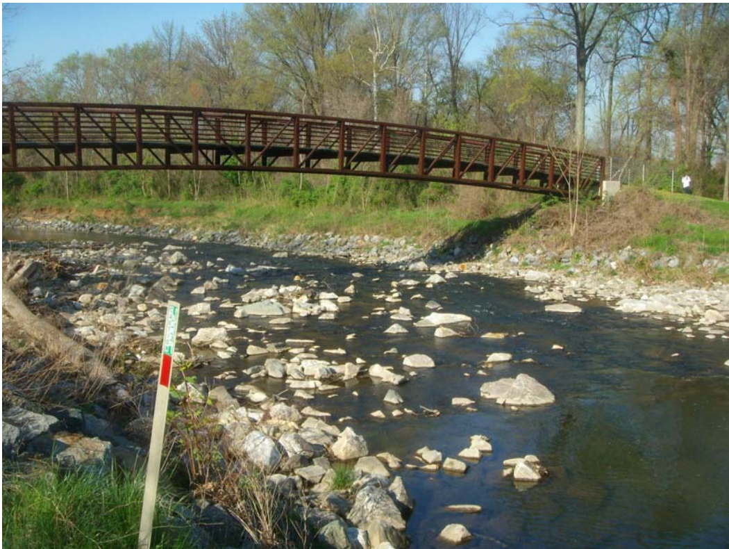
Northwest Branch – 6 looking downstream, April 2008
